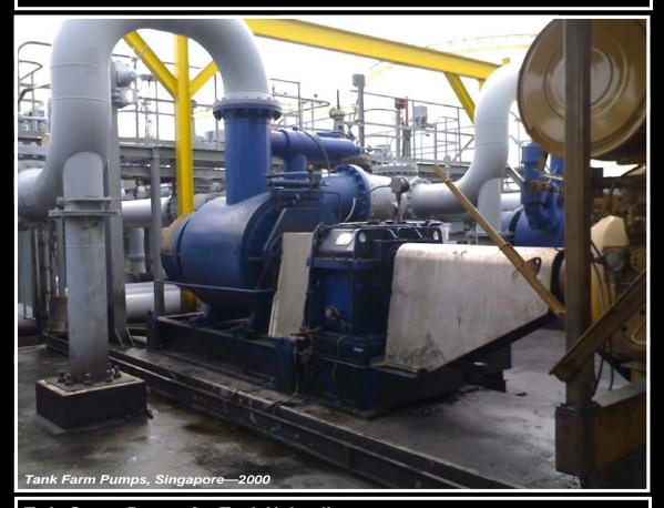
Twin Screw Pumps for Tank Unloading
